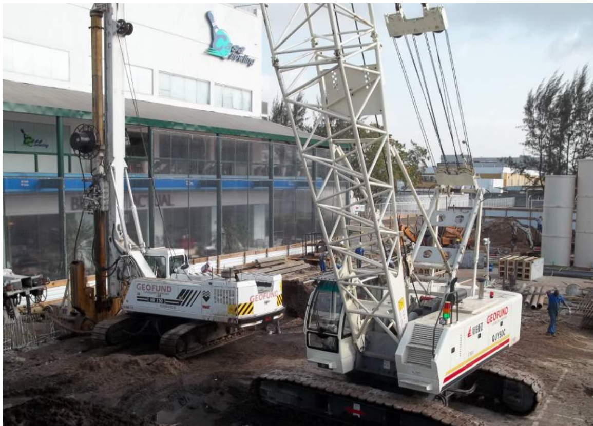
Parede Diafragma Diaphragm Wall
